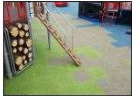
ROOFTOP PLAYGROUND SURFACES: RUBBER TILES DURASOFT TILES THICKNESS PER MAXIMUM CSA FALL HEIGHT STANDARD FOR HIGHEST PLAY ELEMENT COLOURS TBD, ALIGN AT 45 DEG. AS SHOWN, OR SIMILAR PREAPPROVED SUBSTITUTE
