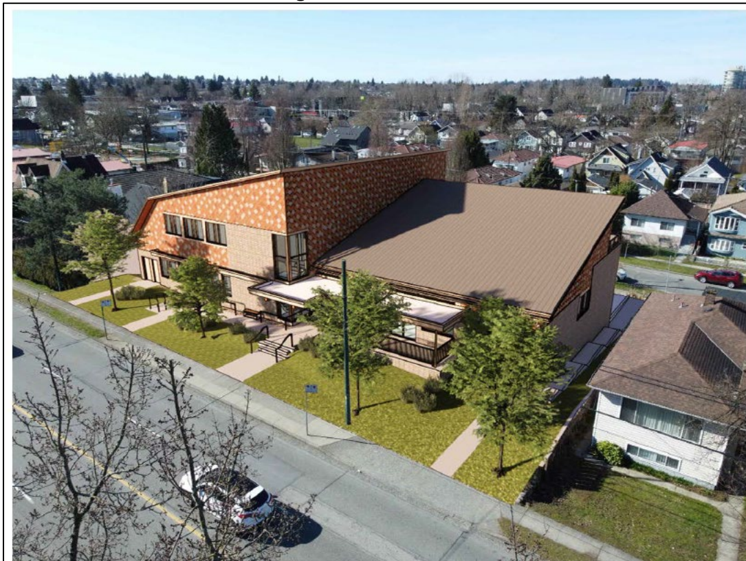
LOOKING SOUTHWEST ON VICTORIA DRIVE
