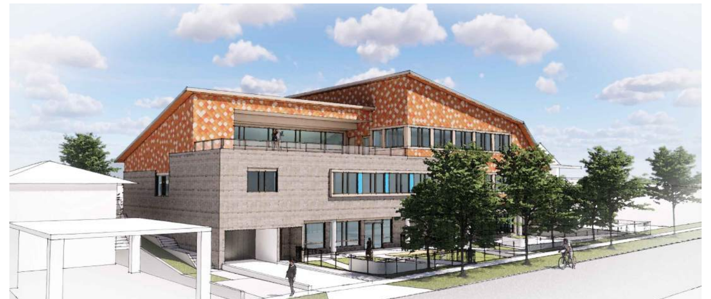
LOOKING SOUTHEAST ON ALICE STREET
