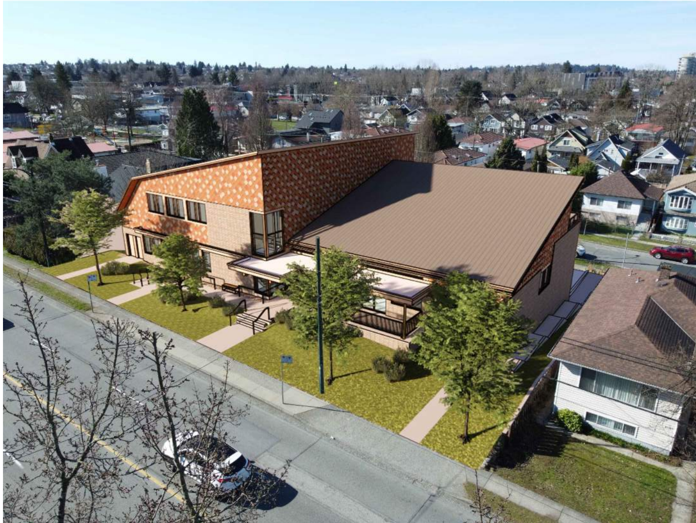
LOOKING SOUTHWEST ON VICTORIA DRIVE
