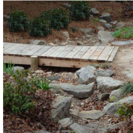
BRIDGE AND DRY STREAM
