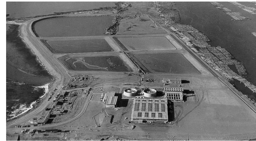
Iona Island Wastewater Treatment Plant – 1963 opening
