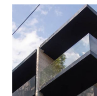
GLASS + ALUMINUM GUARDRAIL
