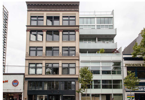
Potential built form example - 47 West Hastings Street
