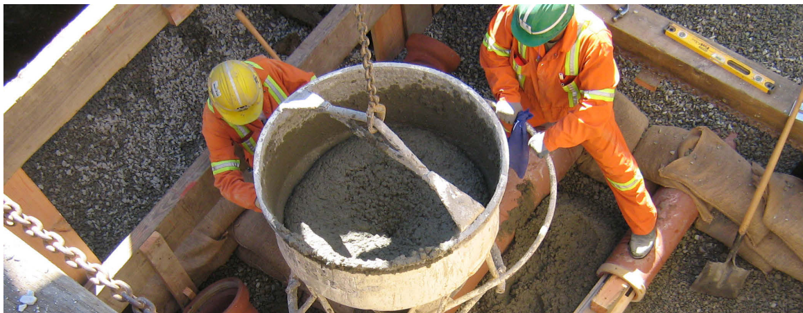
Utility infrastructure maintenance
