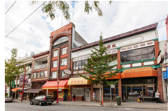
Heritage Society Buildings on East Pender Street in the Chinatown National Historic Area
