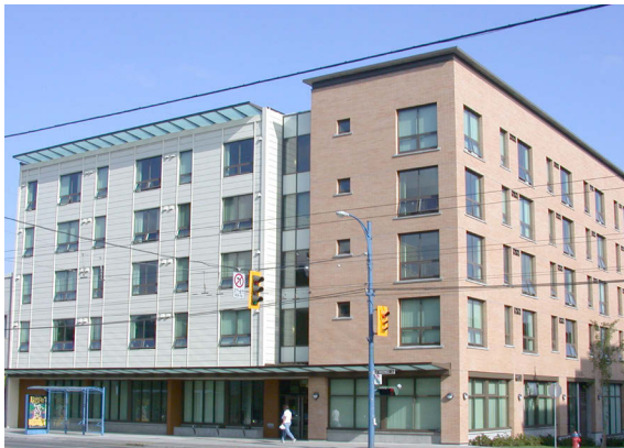
The Smith-Yuen Apartments is purpose-built social housing for seniors, located in the Downtown Eastside Oppenheimer District
