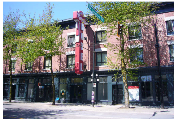
The Rainier Hotel was purchased and renovated by BC Housing, and is managed by a non-profit, to provide housing for marginalised women
