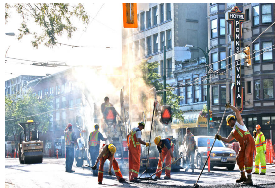
Hastings Street public realm and road improvements
