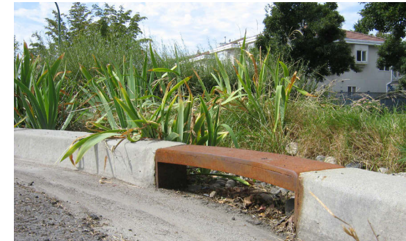
Example of sustainable design elements in the Carrall Street Greenway include storm water infiltration planter boxes, a permeable paver system, and rainwater channels
