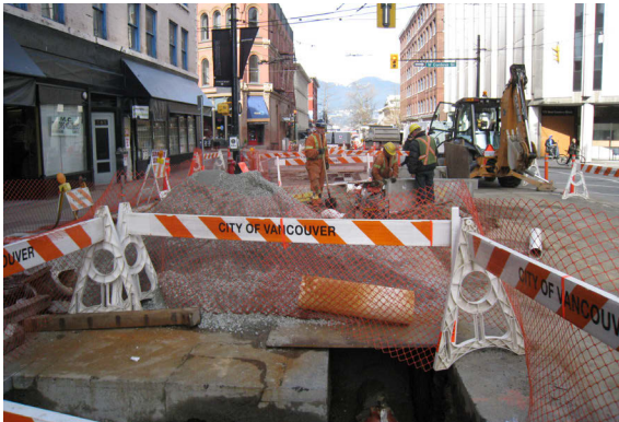
Sewer construction in Gastown
