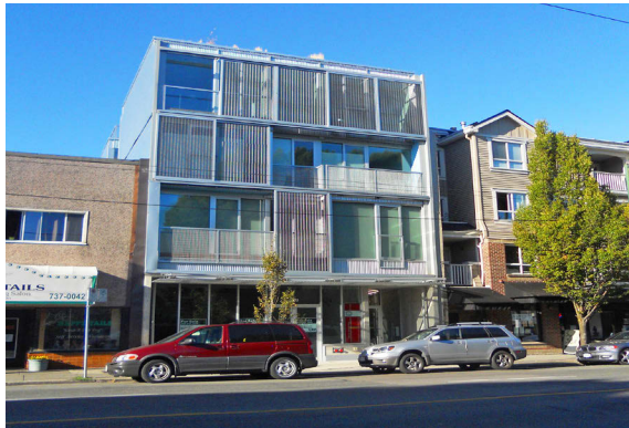
Potential built form - 3351 West 4th Avenue
