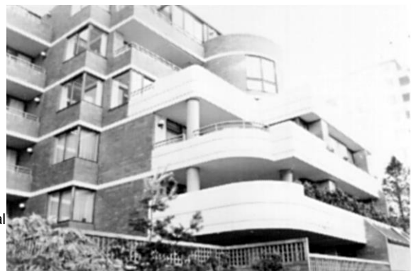
Balconies as a major architectural component of the design.
