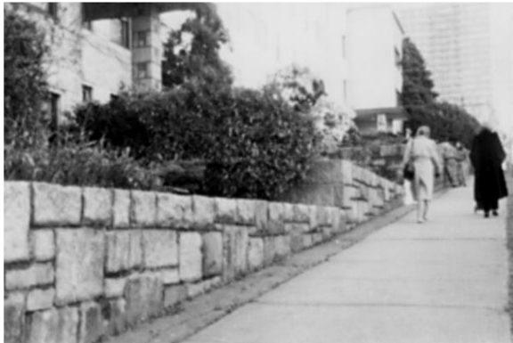
A representative masonry retaining wall.
