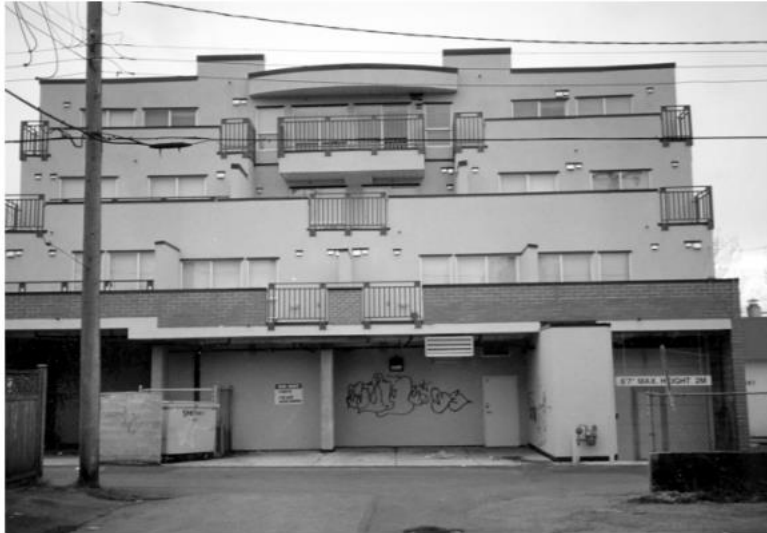
Figure 17: Example of poor treatment of parking and service area off the lane
