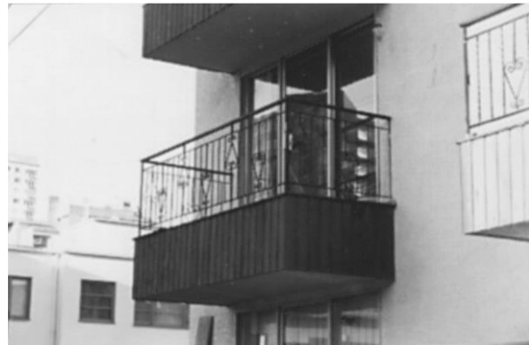
This projecting balcony appears tacked on.
