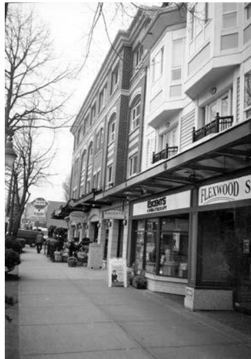
Figure 30: Example of pedestrian-friendly frontage
