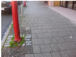
Figure 11. Sidewalk paving pattern and granite cobblestones detail
