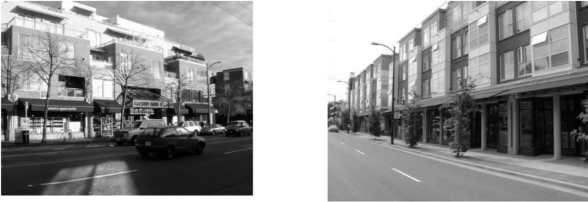
Figure 19: Examples of architecturally integrated, high quality awnings and canopies
