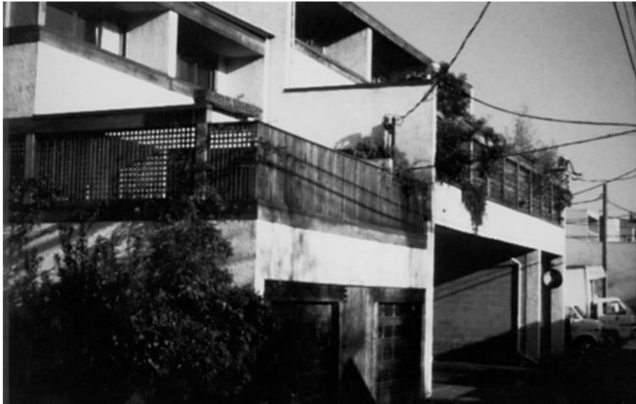
Figure 21. Parking and loading area covered and used for landscaped roof decks
