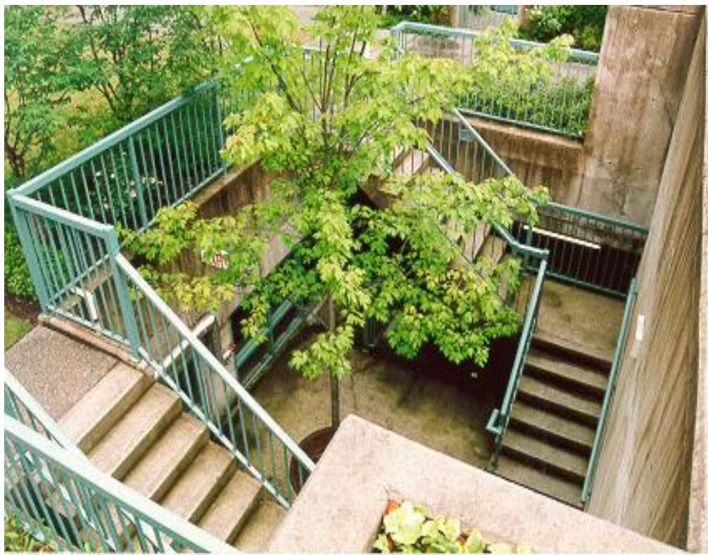
Figure 8. CPTED Exit Stairs
