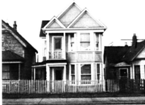
Example of multiple gable roof.
