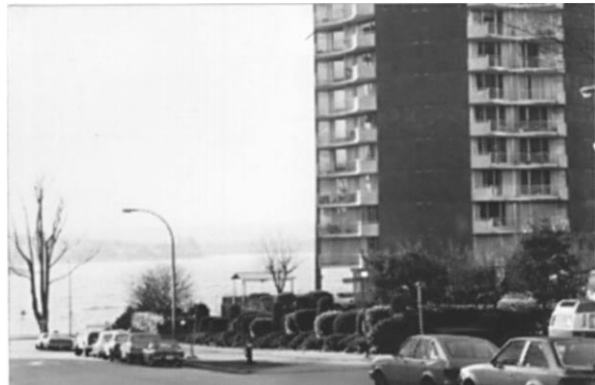
Example of a tower pulled back from the street to create a view corridor.
