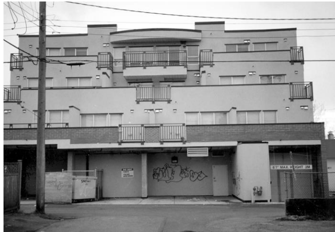
Figure 27: Example of poor treatment of parking and service area off the lane
