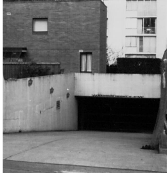
Figure 10. Lack of Quality Treatment of Vehicular and Service Area
