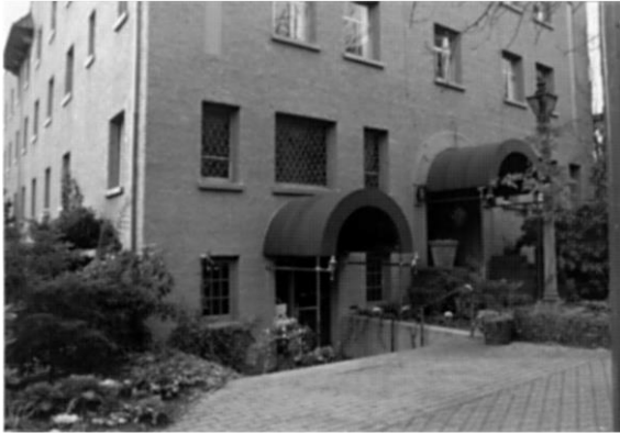
Awnings creating entrance identity and character.
