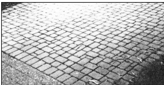
Figure 64. Brick Paver Drive
