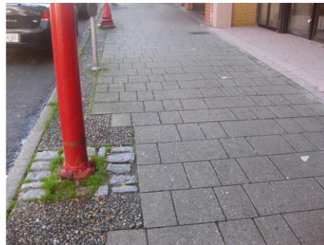
Figure 22. Sidewalk paving pattern and granite cobblestones detail
