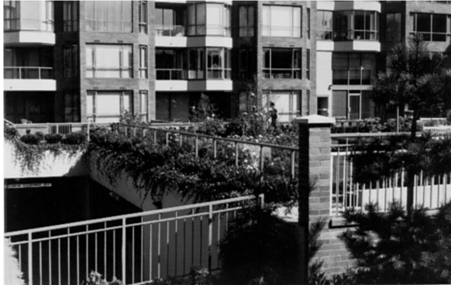
Figure 36. Parking entrances and roof decks are improved through high-quality landscaping
