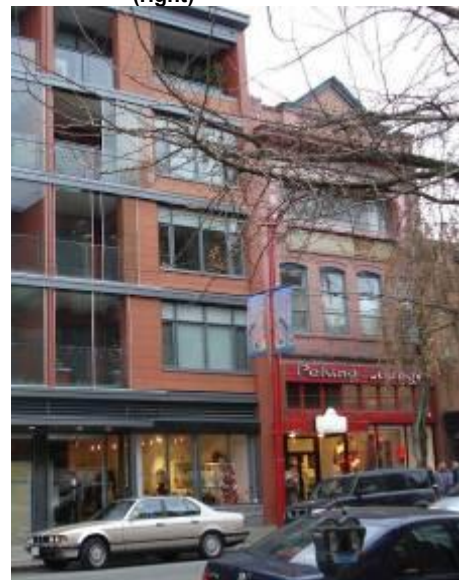
Figure 2. Compatible contemporary building (left) adjacent to heritage building (right)
