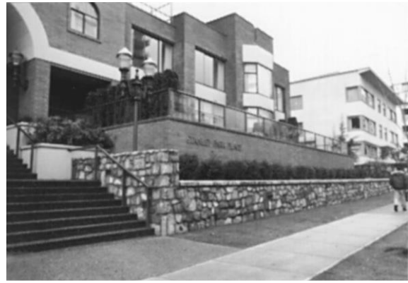
Retaining wall stepped to respond to topography.
