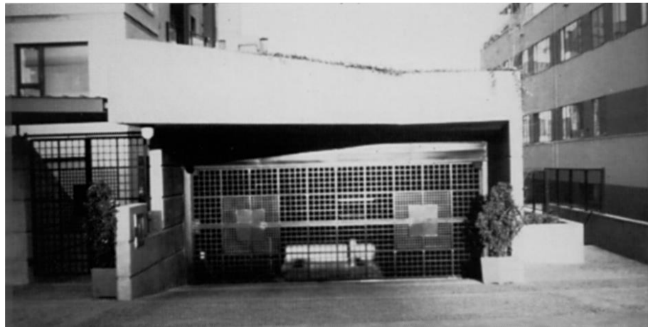
Figure 23. Well-designed and screened service areas improve lane quality
