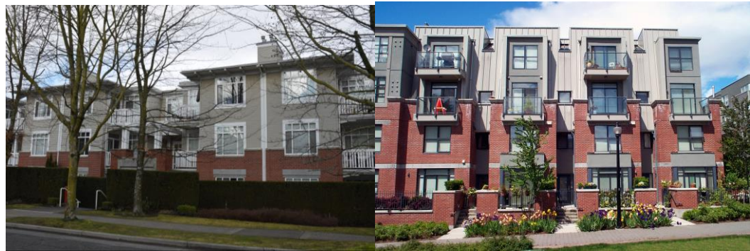
Figure 12: Varied rooflines on multiple dwellings
