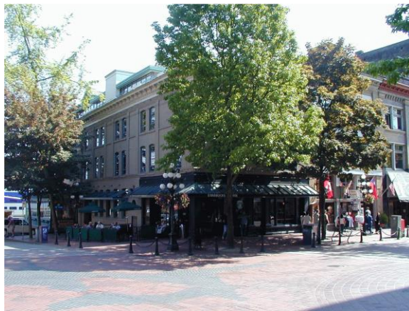
Figure 5. Addition to existing building
