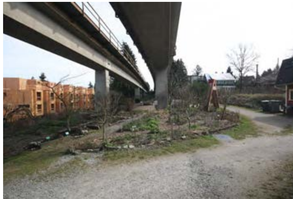
EAST VIEW UNDER SKYTRAIN GUIDE-WAY
