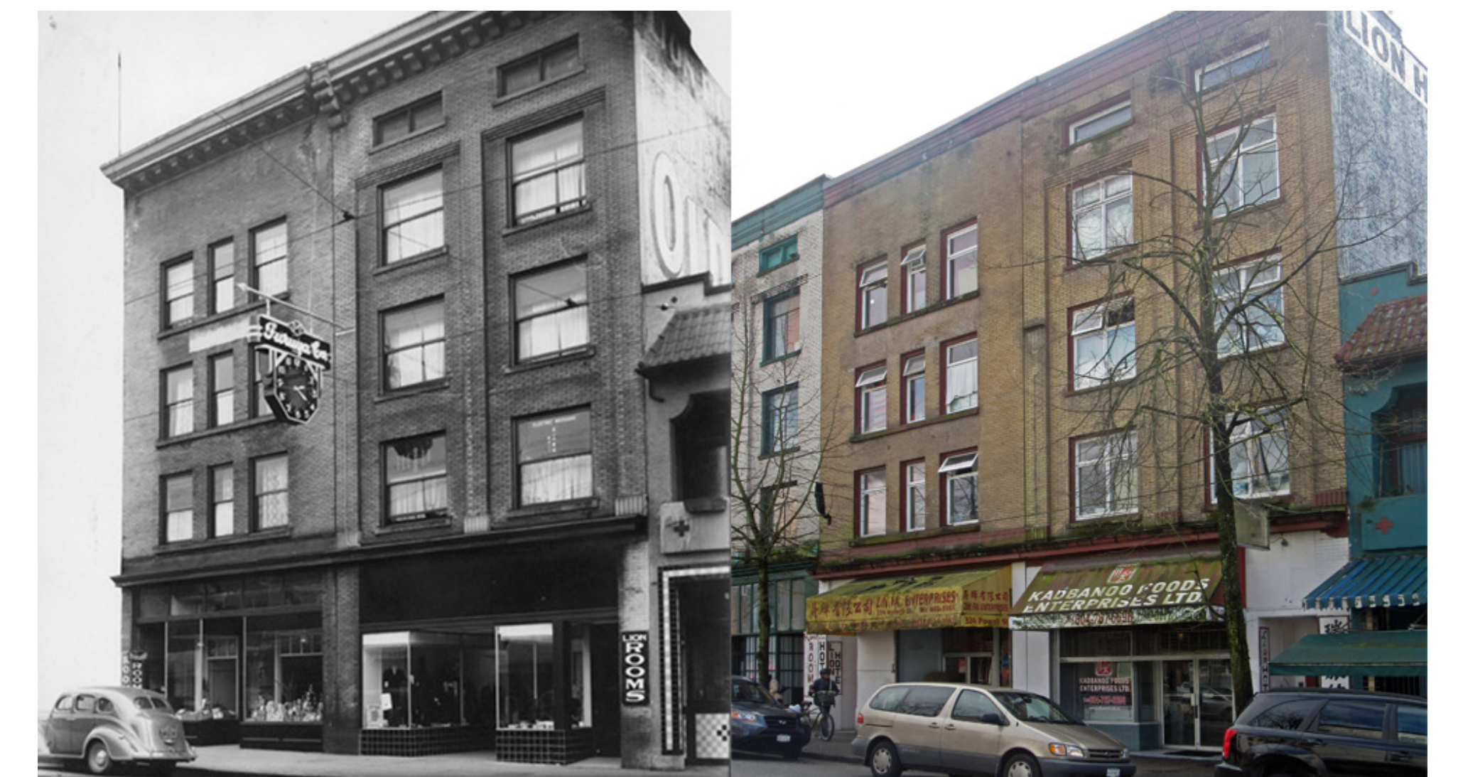
Brick and Tile at 318 & 324 Powell Street
