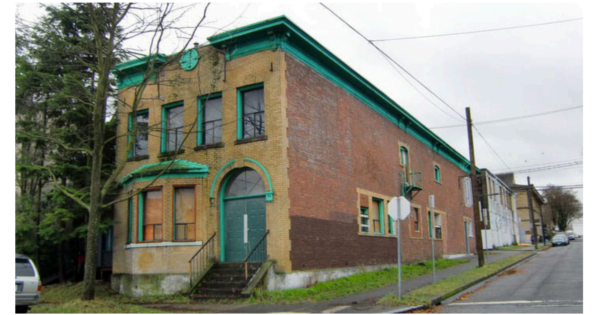
Brick facade of 1912 building at 500 Alexander Street
