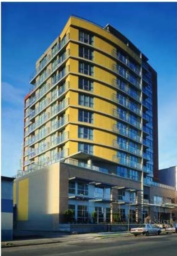
Figure 3 Seymour Place and Coast Mental Health Resource Centre - Yaletown -136 units Opened 2000
