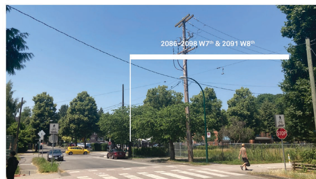
3 View of 2086-2098 W7 th & 2091 W8 th from 8 th Avenue at Greenway (looking North-West)
