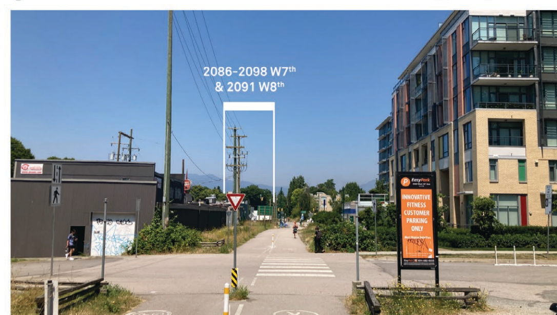
5 View of 2086-2098 W7 th & 2091 W8 th from 10 th Avenue at Greenway (looking North)
