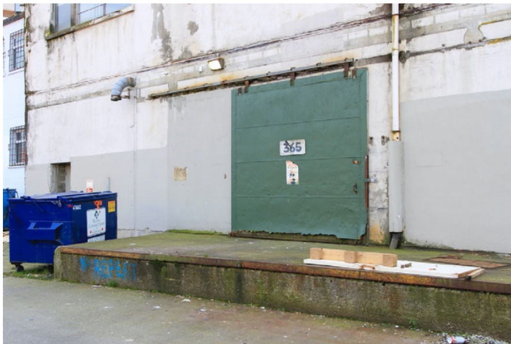
Detail photo showing original sliding door and raised platform.
