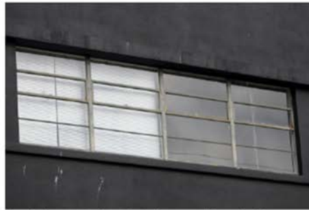
Detail of an original metal window assembly on the front elevation of the Fleck Brothers Warehouse.
