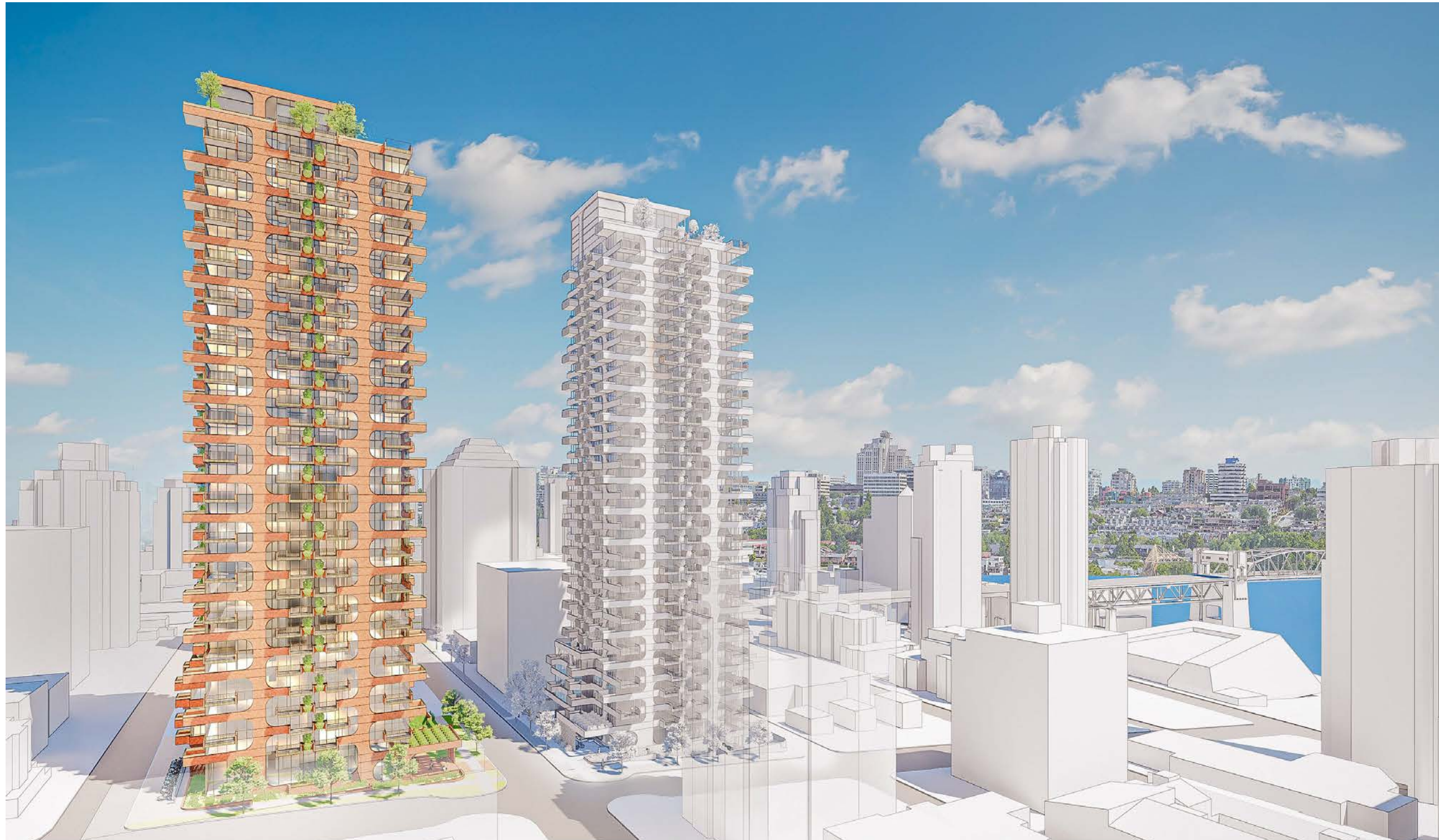
View from Harwood Street looking South
