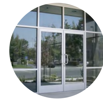
3 Clear curtainwall / storefront glazing
