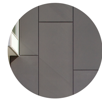
2 Pre-finished metal cladding
