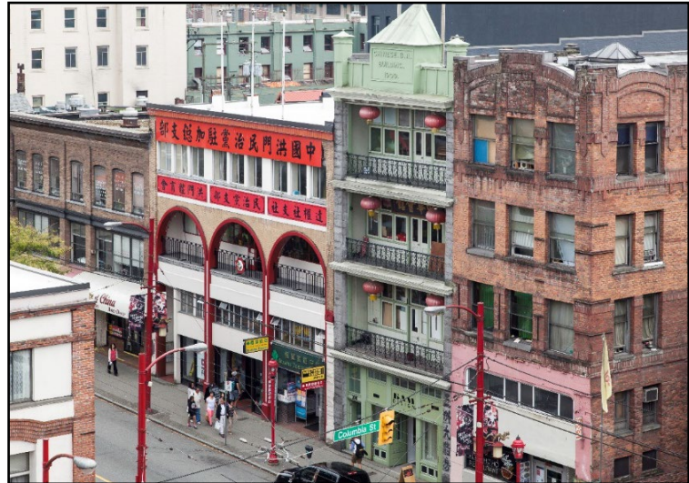
Figure 9: 100 Block Pender Street East
