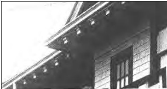
Figure 34. Flat Soffit
