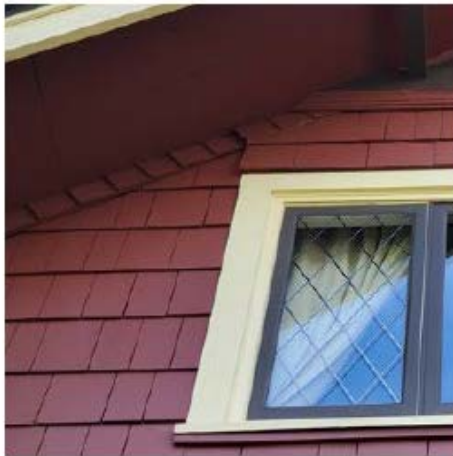
Existing roof overhang with unsympathetic plywood soffit. Note shingle frieze band at soffit-to-wall interface.
