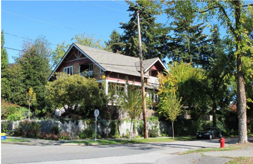
Figure 2: Prior to maintenance work
