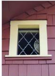
Original single-glazed, leaded wood window sash (upper floor)
