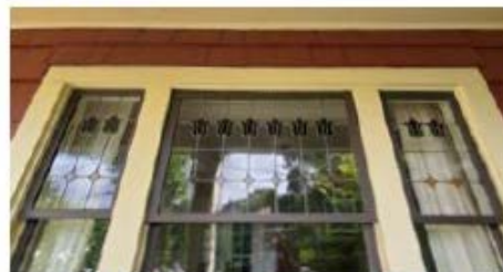
Tripartite double-hung wood window assembly at verandah (facing East 6th Avenue).
