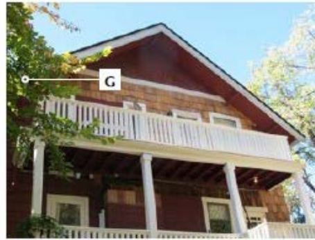
Rear elevation: showing replacement of wood shingles in 2017.
