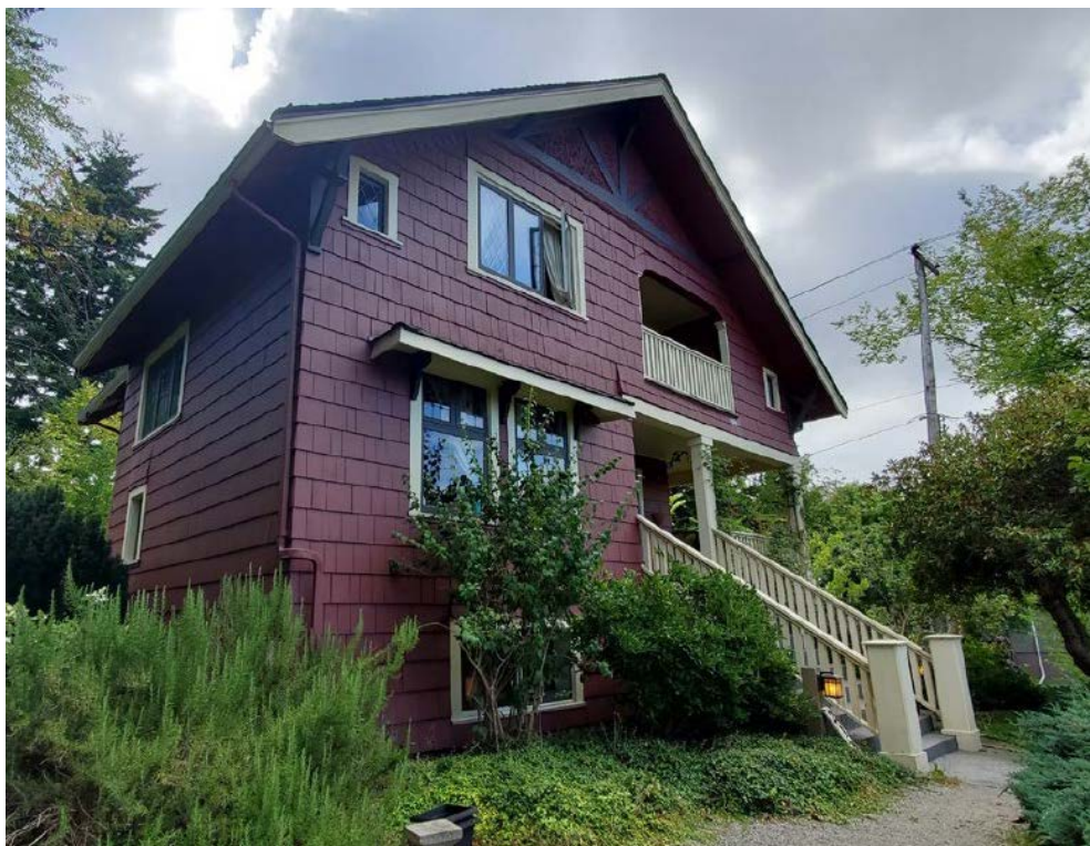
Figure 3: After maintenance work (e.g. repainting, roof repairs, select replacement of window assemblies)
