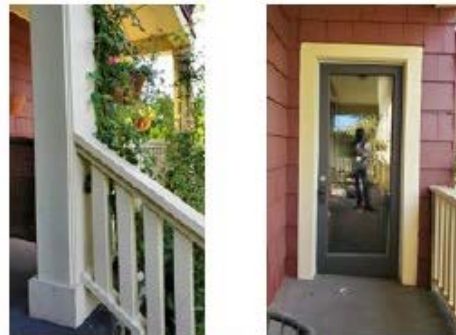
Left: Existing square column and open balustrade. Right: Existing secondary door opening with replacement door, located at return of verandah to the south.
