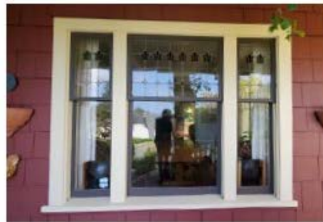
Tripartite double-hung wood window assembly at verandah (facing Semlin Drive).
