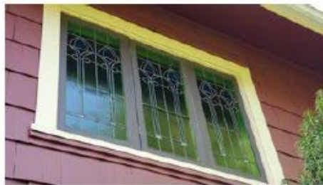
Side (north) elevation: original tripartite wood window assembly at upper level.
