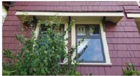
Front elevation: original paired wood window assembly.
