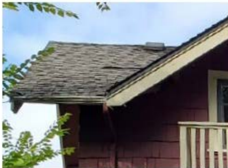
Photo showing existing roof cladding and trims. Note contemporary roof vent along ridge of gable dormer.
