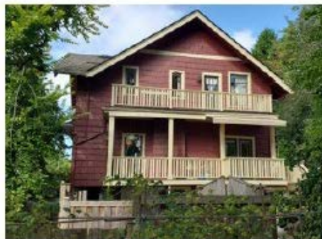
Rear (east) elevation. Note porches on main and upper floor levels that are not original.
