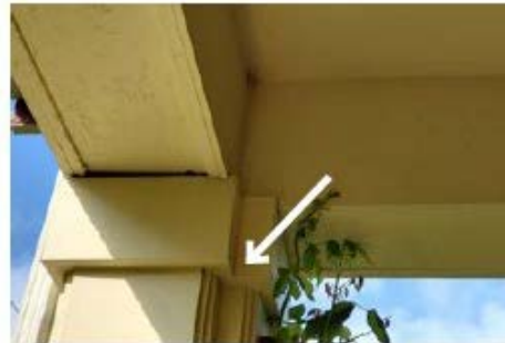
Detail photo showing column cladding details that are not historically appropriate.
