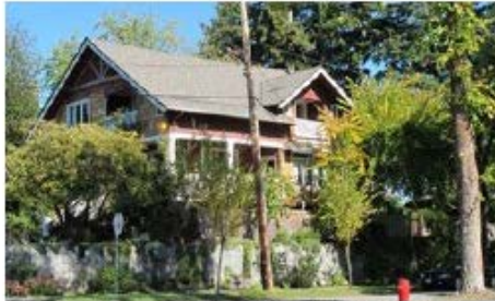
Photo showing primary gable roof structure and projecting dormer.
