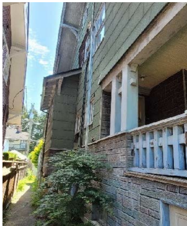
Detail photo of partial east elevation, showing existing bay window proposed to be altered to introduce new entrance to a separate dwelling unit. (Photo credit: Julie Schueck)
