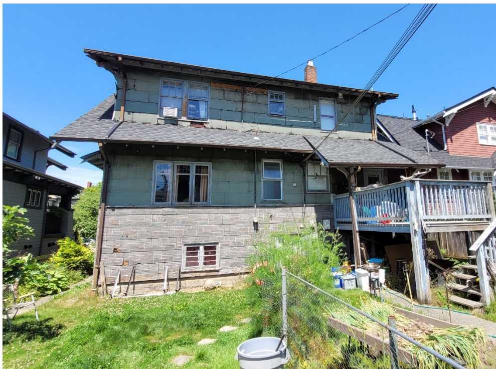
South (rear) elevation. (Photo credit: Julie Schueck)
