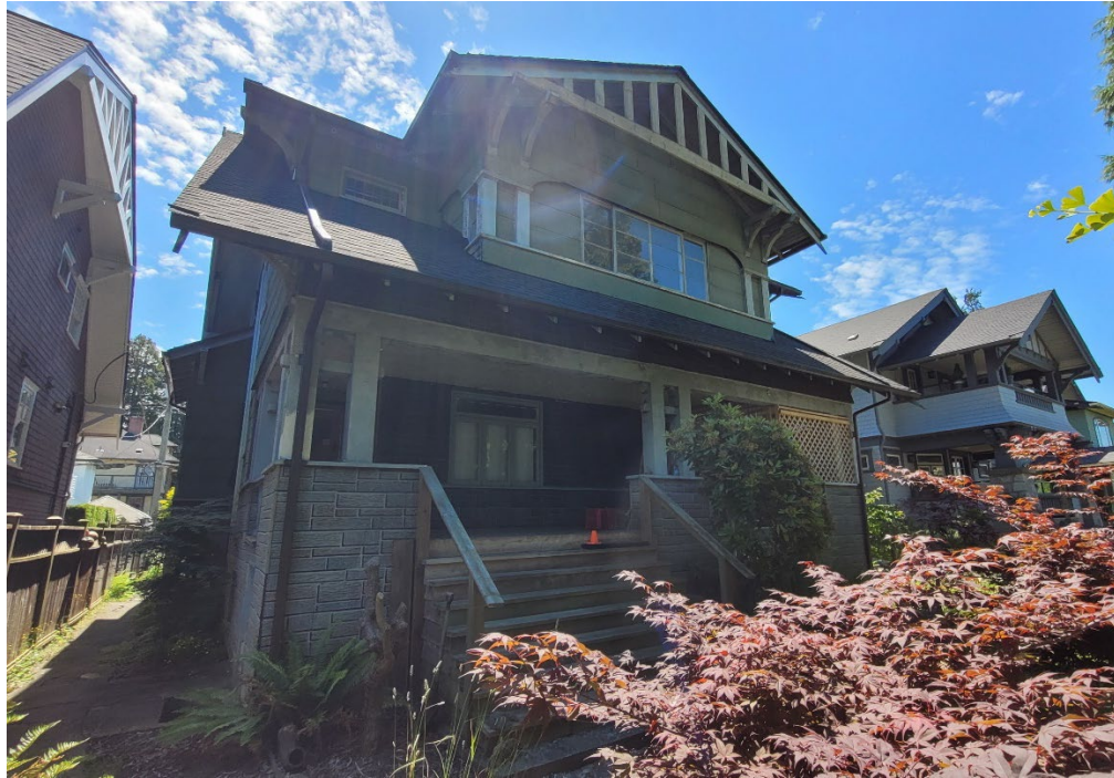
North elevation, showing partial east elevation. (Photo credit: Julie Schueck)
