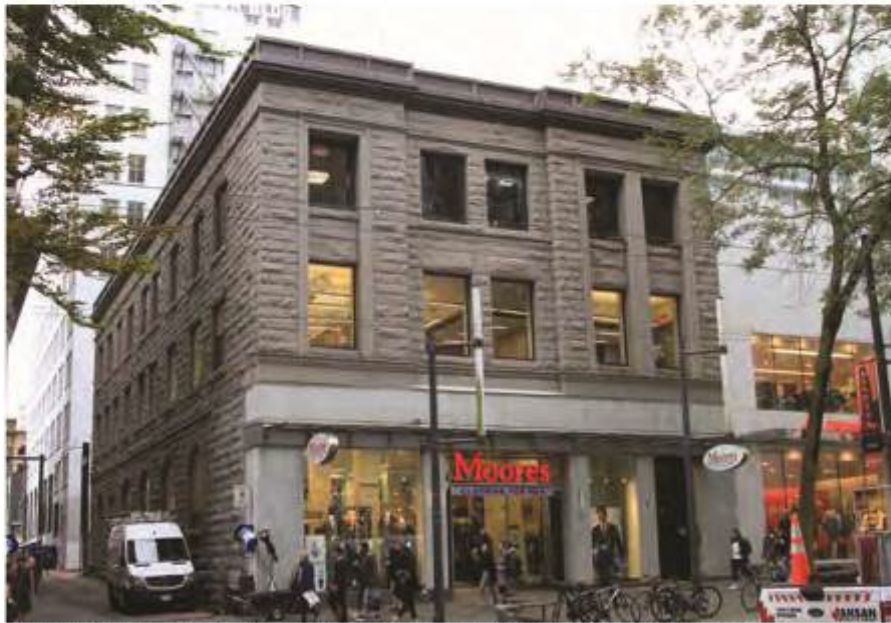
Above: Three-storey Leckie Block with rectangle plan, stone construction, flat roof behind parapet. Front façade shows three structural bays with recessed middle bay. Storefront and parapet cornice are later interventions.
