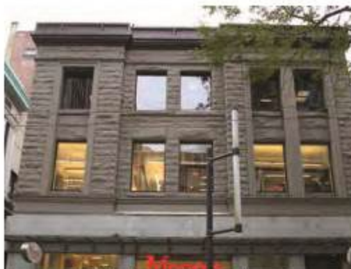
Above: Single and double assembly rectangle window openings on front (northwest) façade. All windows on the building have been replaced.
