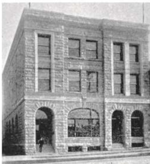
Above: Original equal 1-over-1 wood windows present on second and third floors of the front (northwest) façade.
