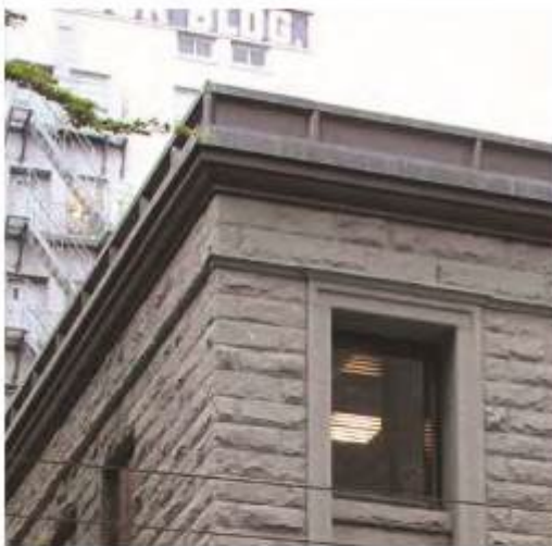
Above: Later installed metal cornice and flashing concealing original parapet, cornice, and coping.
