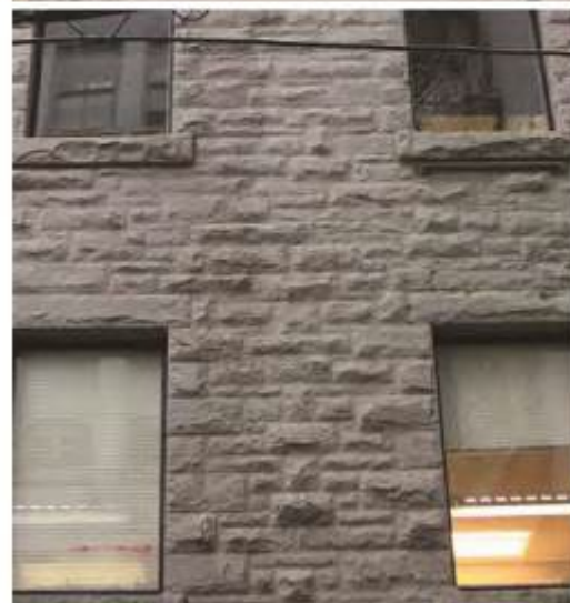
Above (top): Sandstone exterior of front (northwest) and northeast laneway façades laid in block course.
