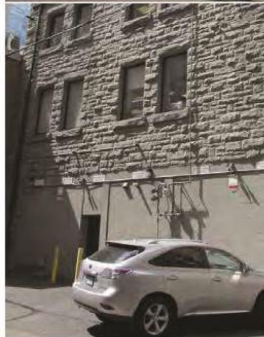
Right Bottom: Alterations to ground floor of rear façade with openings resized and infilled with concrete block.
