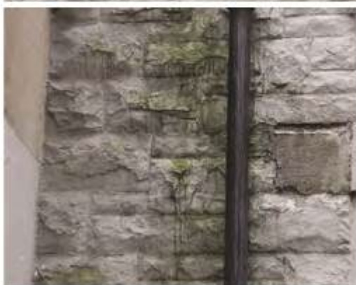
Above: Examples of typical deterioration including: delamination where sandstone is exposed behind later applied paint (top); staining (middle); and organic deposits and saturated stone (bottom).
