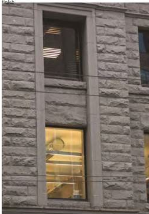
Below: Window surround present on front façade. Sandstone sills and lintels and continuous drip mould band with tooled finish.
