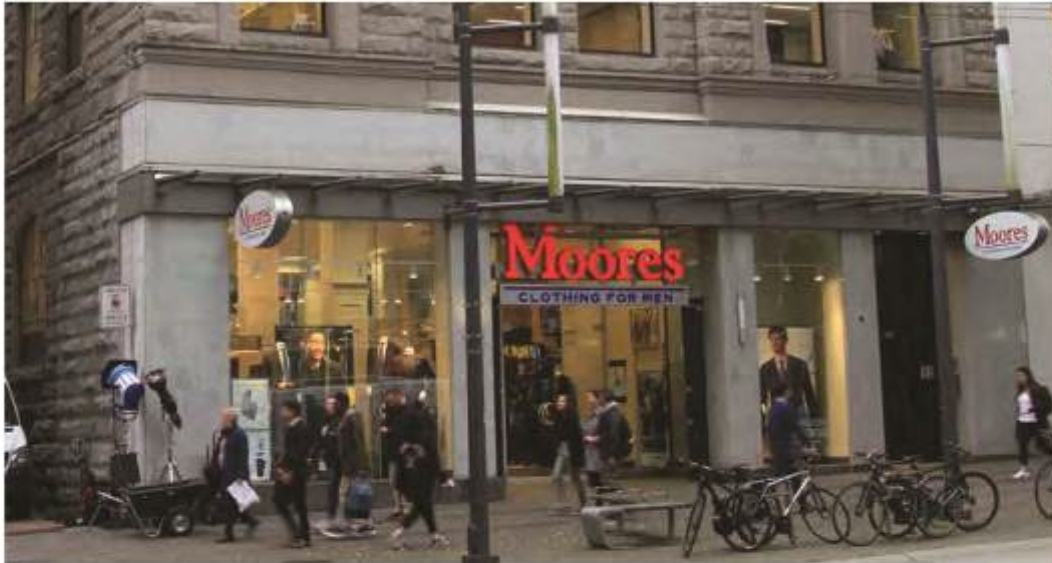
Above: Current appearance of Leckie Block storefront with northeast laneway façade infilled and clad in granite rockface veneer. Polished granite tile on the front façade, full-height glass storefront, and glass and metal canopy. The storefront cornice is partially intact except for the bullnose course at the bottom of the cornice.
