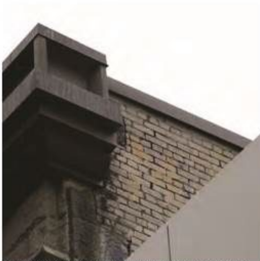
Above: Brick façade of party wall laid in common bond with mortar loss evident.
