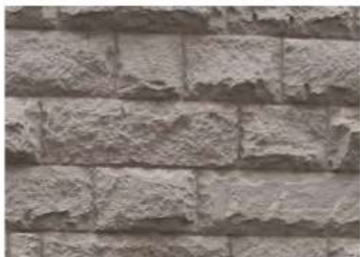
Above: Rusticated stone units with rockface finish.
