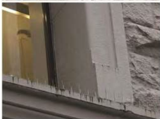
Above: Examples of typical deterioration including: delamination where sandstone is exposed behind later applied paint (top); staining (middle); and organic deposits and saturated stone (bottom).
