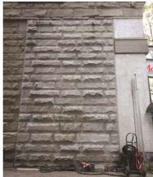
Right Top: Later installed granite on northeast laneway façade where storefront extension was filled in.
