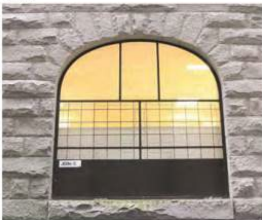
Above: Basket-handle window openings present on ground floor of northeast façade with sandstone voussoirs, sill, and replacement window. Organic deposit present on multiple sills on building.
