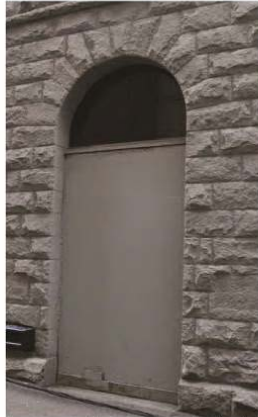
Above: Intact original door opening on ground floor of north façade with sandstone voussoirs, transom has been replaced, and door boarded over.
