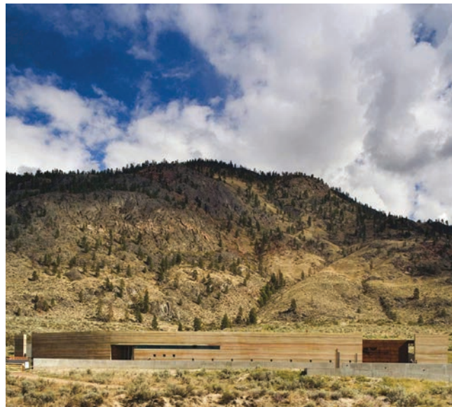
Figure 8-64: NK'Mip Desert Cultural Centre, Integrate Building with Landscape
