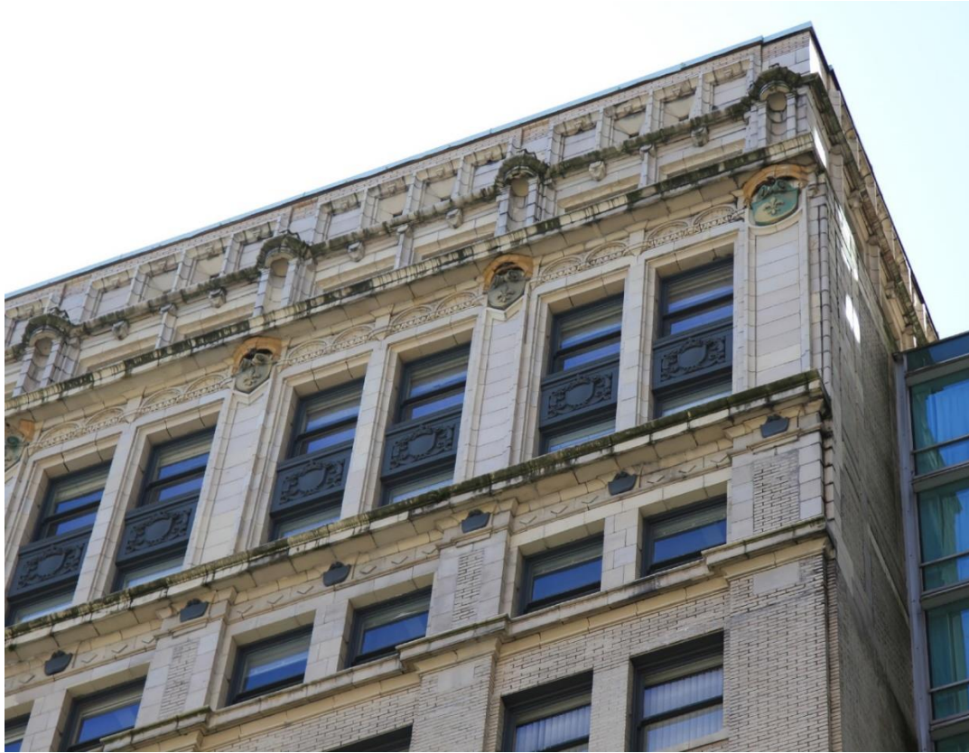
Detail photo showing brick and terra cotta elements at upper level.
