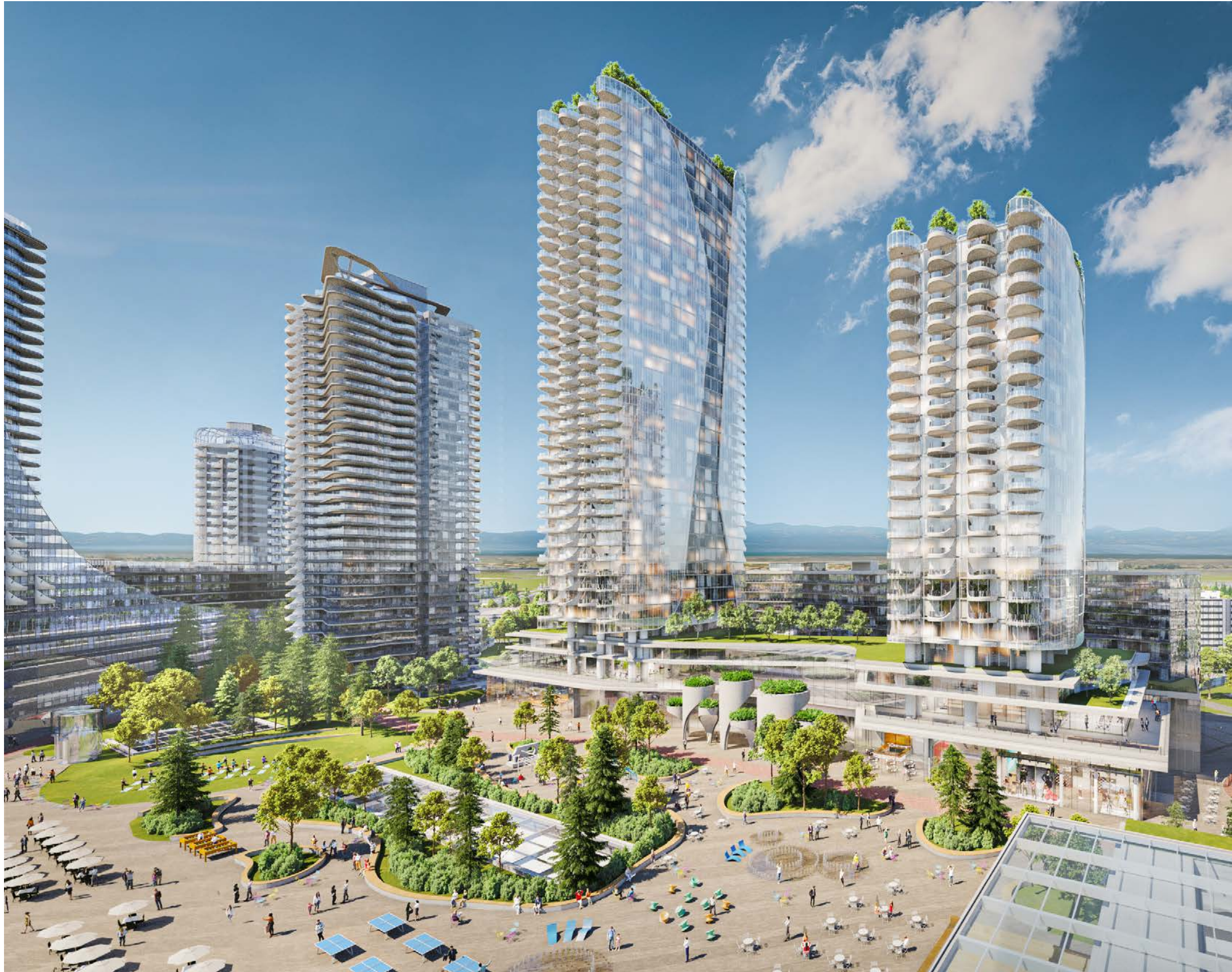
View of Buildings 13 and 14 from The Commons looking South
