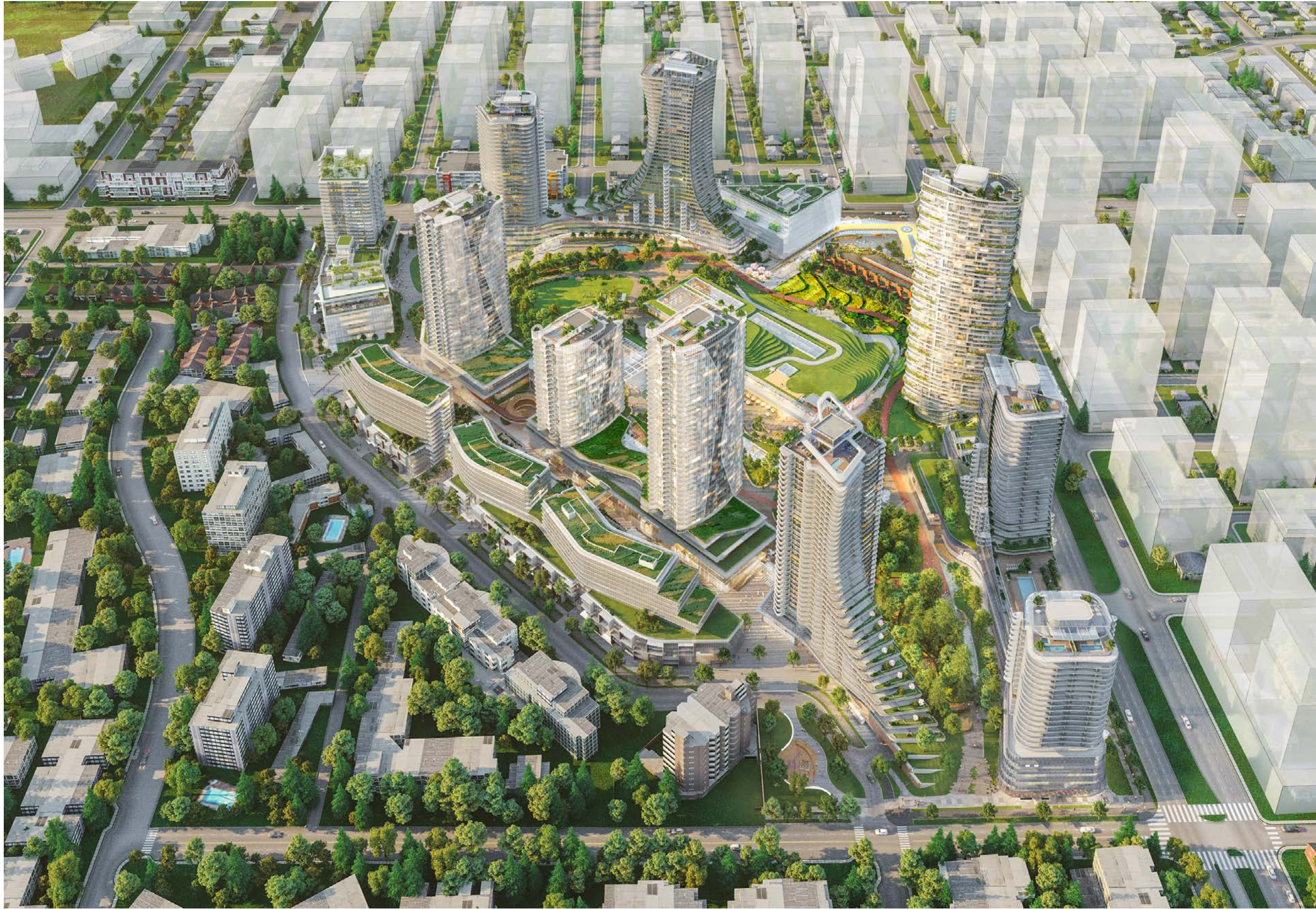
Aerial View looking North
