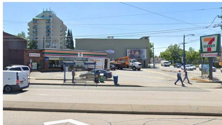
7 - SUBJECT SITE FROM KINGSWAY
