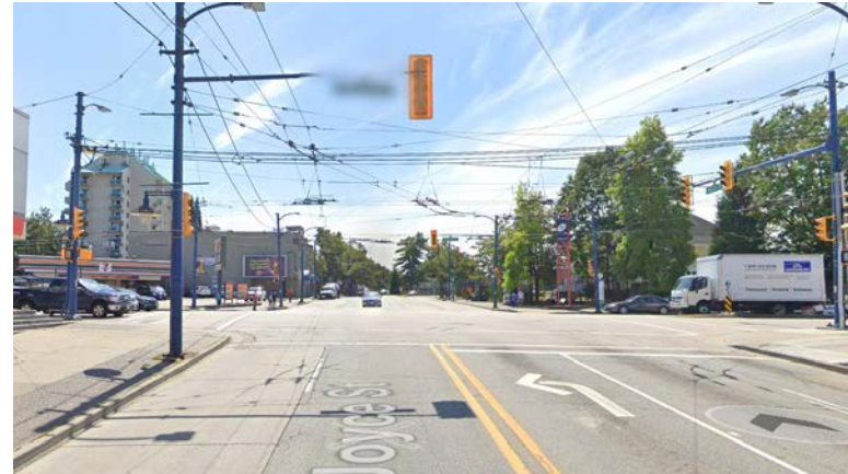
2 - ALONG JOYCE STREET TOWARDS SOUTHWEST
