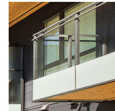
GUARDRAILS CLEAR GLASS W/ FROSTED BAND
