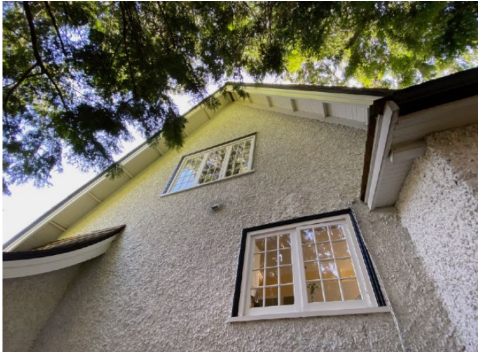
Photo 2: North side elevation of 6237 Adera Street
