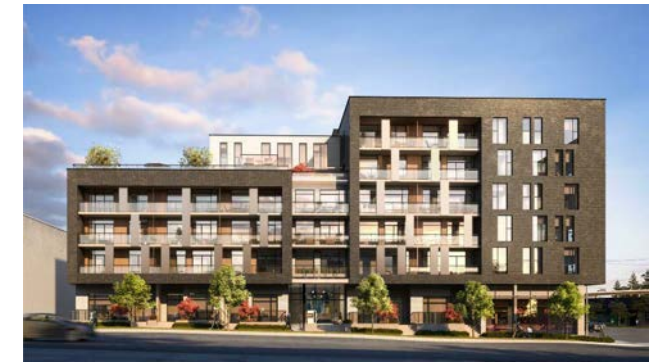
8 - 8888 OSLER (UNDER CONSTRUCTION)
