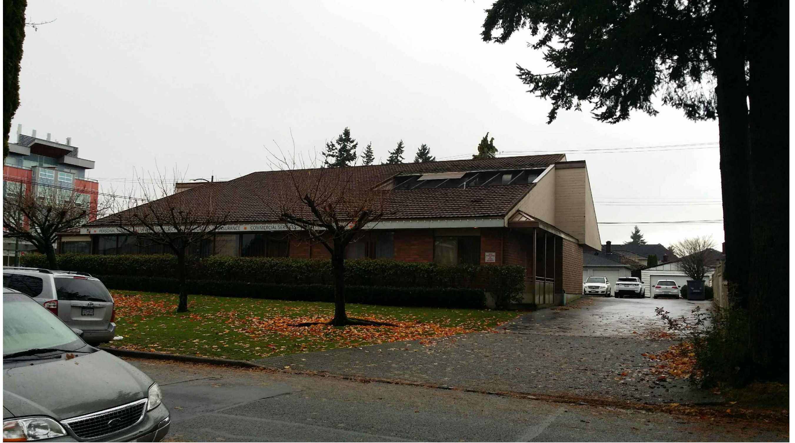
PHOTO LOOKING WEST ON RHODES STREET OF EXISTING BUILDING
