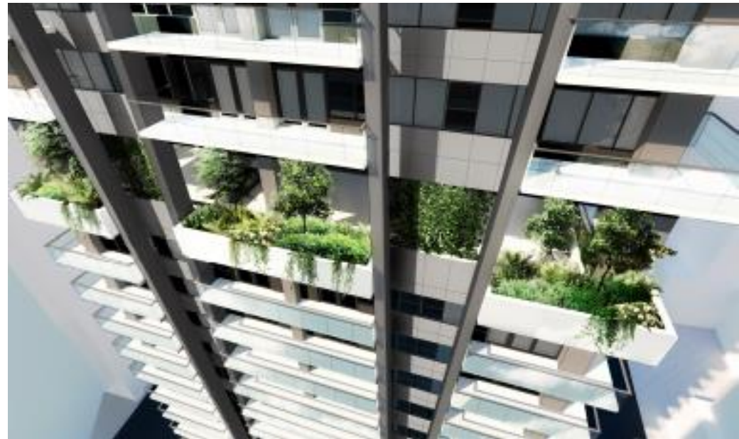
Mid-tower amenity area and building façade
