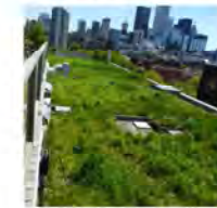
GREEN ROOF PLANTING
