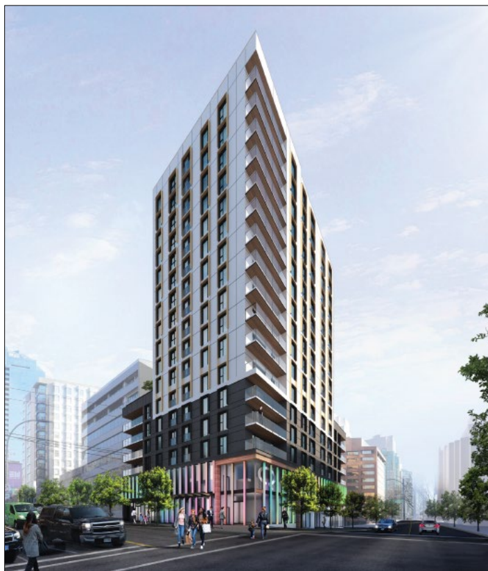
Figure 2: Rendering of Proposed Building from the corner of Burrard Street and Davie Street (looking north-east)
