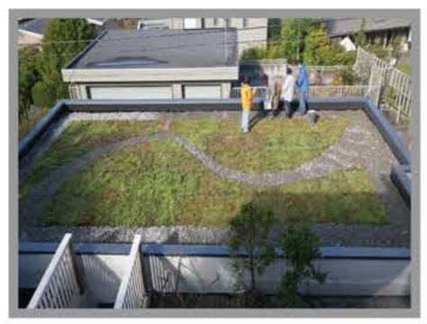
Extensive Green Roof Installation
