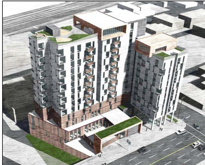
Figure 4: Proposed development: Two wings at different heights, configured in an L-shaped footprint.
