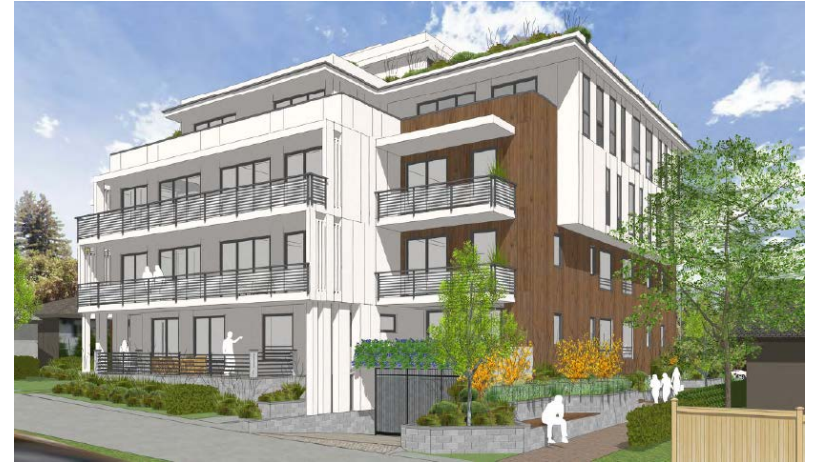
Looking northwest from lane
