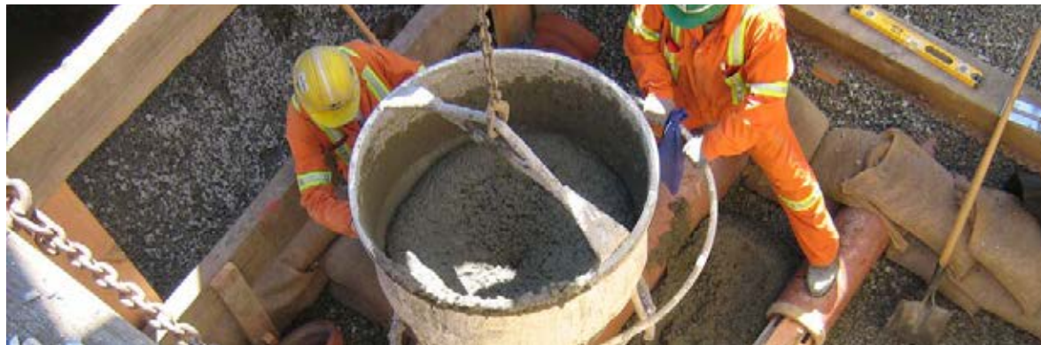
Water main work
