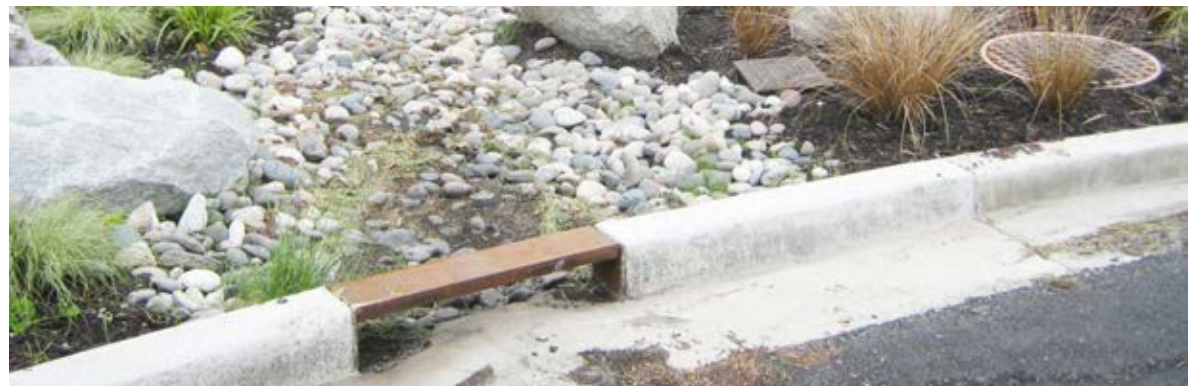
Rain gardens are planted areas behind curbs that filter stormwater from the street
