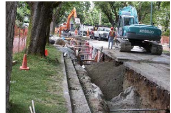
Water main construction
