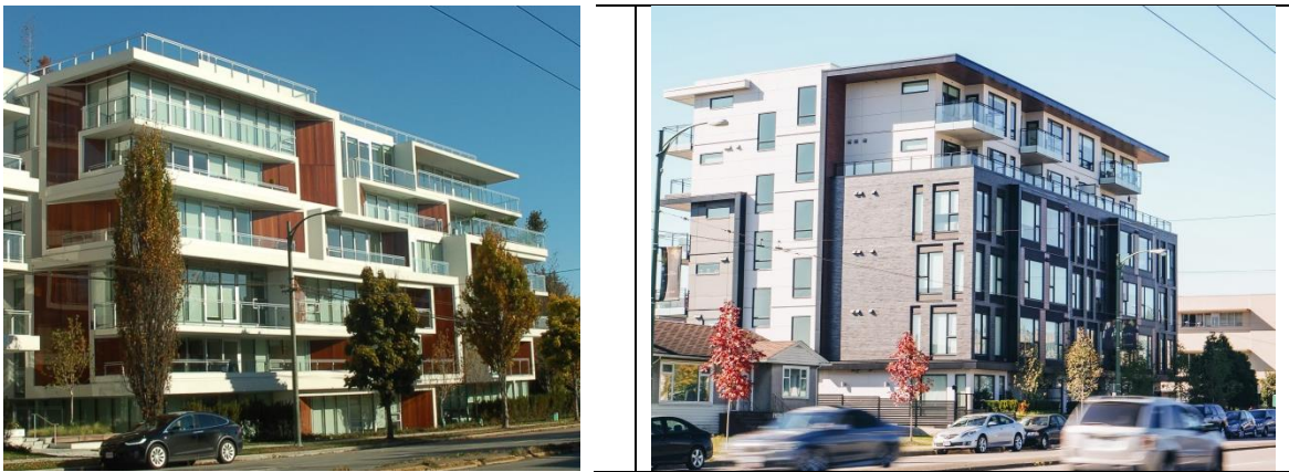
Figure 7: Varied rooflines on multiple dwellings
