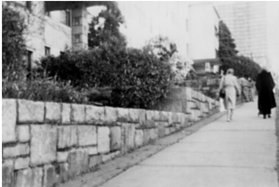
A representative masonry retaining wall.
