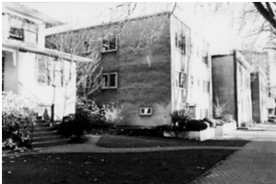
A blank, flanking wall extending beyond the adjacent building is very prominent and requires special attention.
