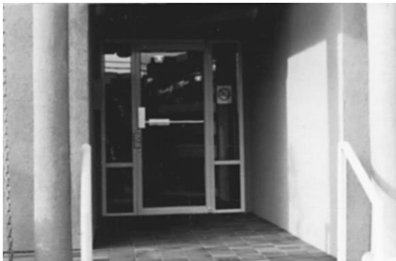
An entrance with limited character and appeal.
