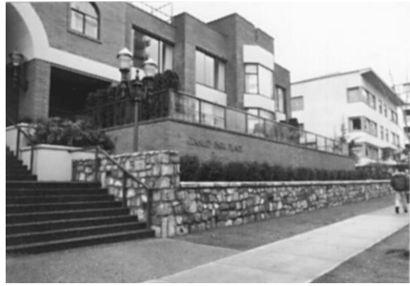
Retaining wall stepped to respond to topography.
