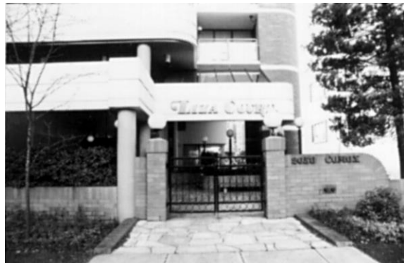
A gateway defining the entrance.
