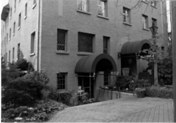
Awnings creating entrance identity and character.
