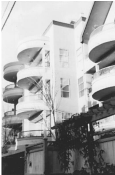
The projecting curved balconies create identity for a building with simple massing.
