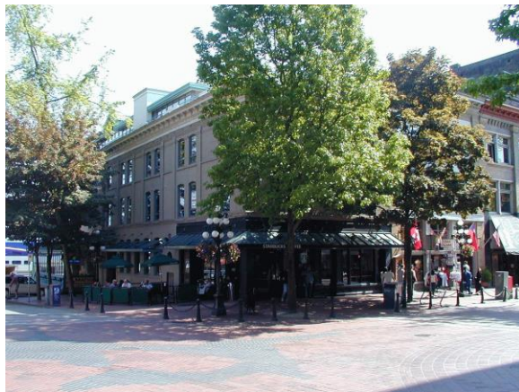
Figure 5. Addition to existing building
