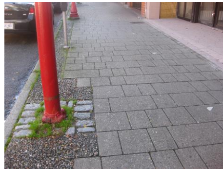
Figure 22. Sidewalk paving pattern and granite cobblestones detail
