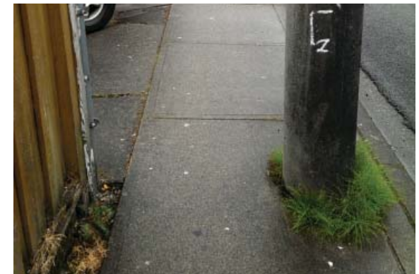
Limited sidewalk space
