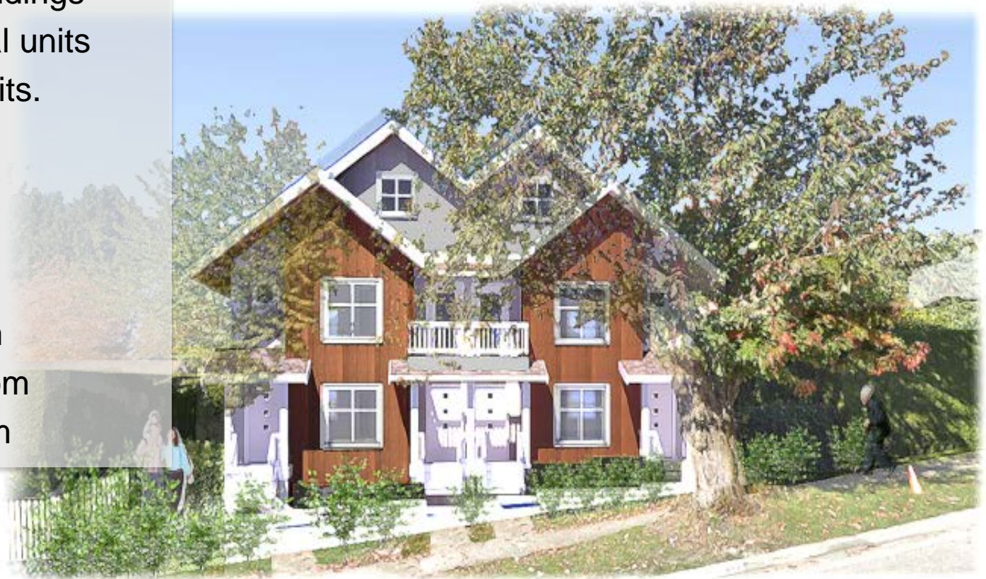
Front View From Dunbar Street
