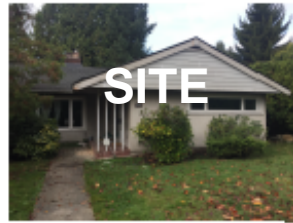
EXISTING HOUSE ON SUBJECT SITE
