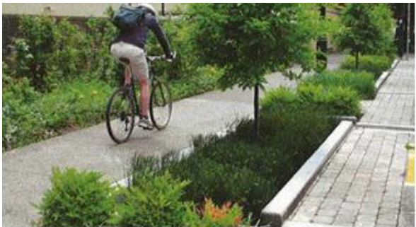
SIDEWALK BIOSWALE TRENCH
