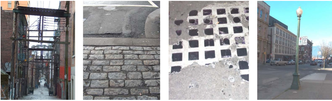
Figure 8-12: Alley H-Frames; Hamilton Street Paving; Areaways; Lamppost
