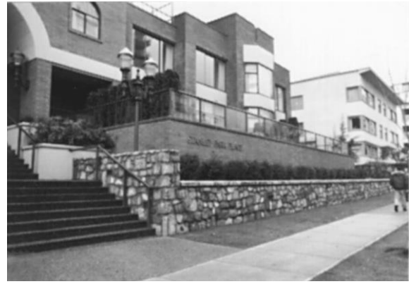
Retaining wall stepped to respond to topography.
