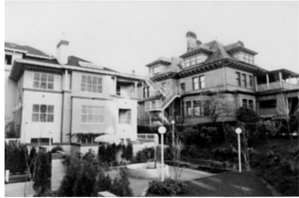
A new building emulating the style and massing of its heritage neighbour.
