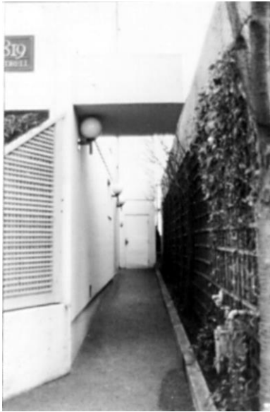
A main access route that is dark, inhospitable and uninviting.
