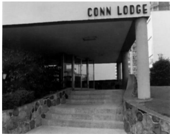
Example of a clear and direct access route from the street to the lobby.
