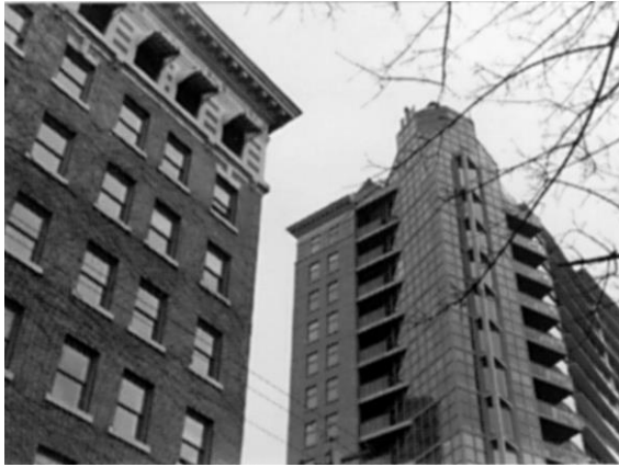
A contemporary building incorporating elements from the adjacent heritage building.
