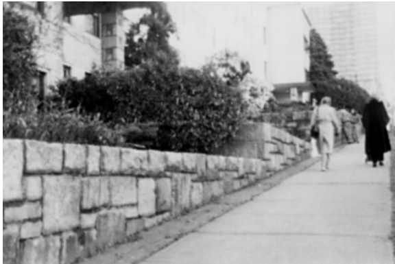
A representative masonry retaining wall.
