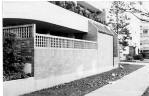
A high blank, wall along the street edge creates an inhospitable image.
