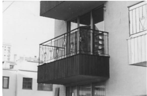
This projecting balcony appears tacked on.
