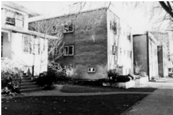
A blank, flanking wall extending beyond the adjacent building is very prominent and requires special attention.
