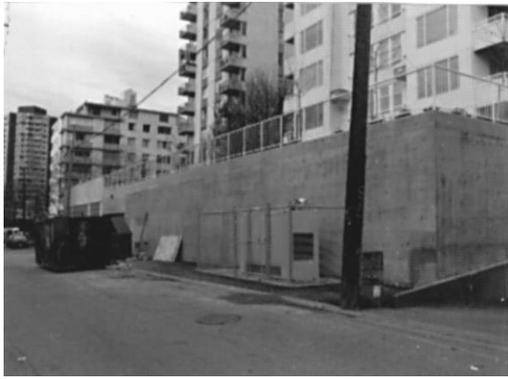
A poor response to topography resulting in an inhospitable image along the lane.
