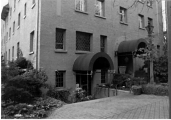
Awnings creating entrance identity and character.
