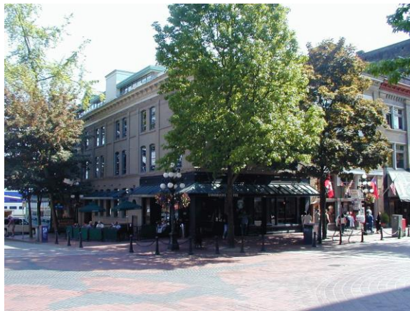
Figure 5. Addition to existing building
