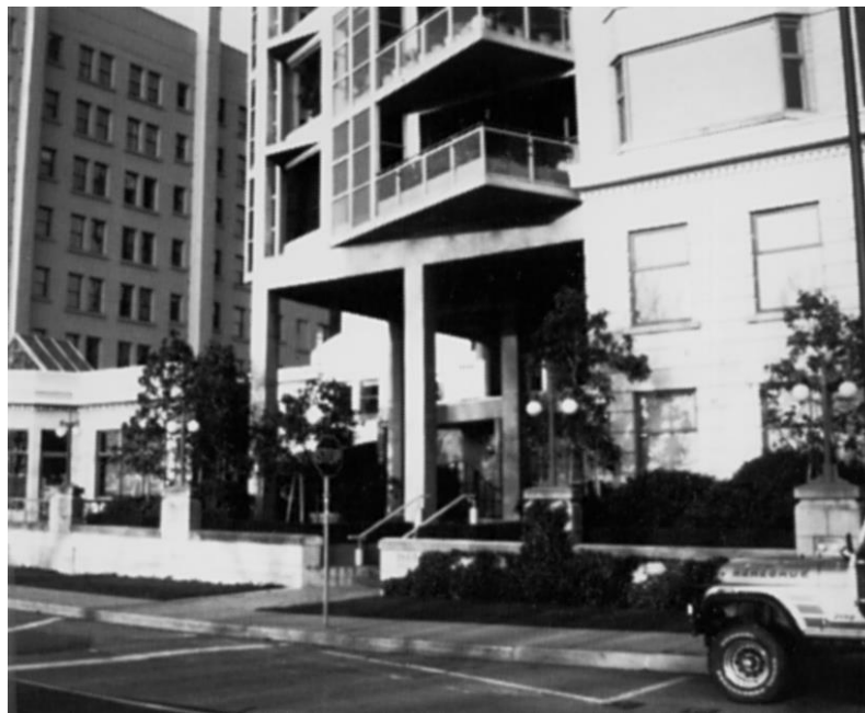
Figure 35. Quality landscaping along the street helps create “residential character”
