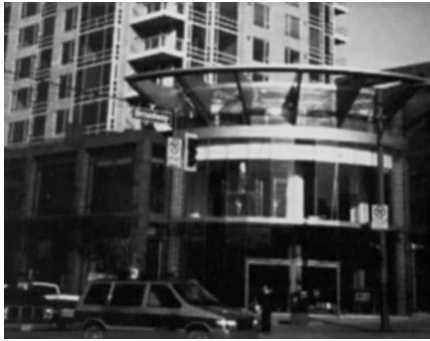
Figure 26(a). Good example of lower level commercial treatment
