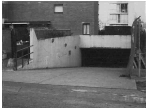
Figure 13. Lack of quality treatment
