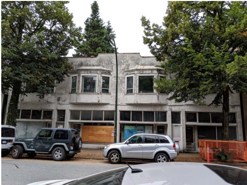
3495-3505 Commercial Street – Front Façade (Current)
