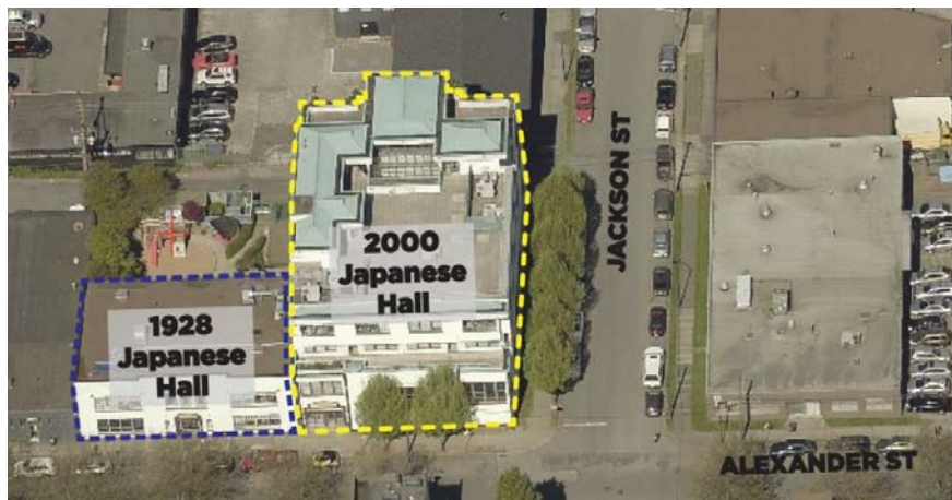
Figure 2 – Aerial view showing the two buildings, the 1928 Building and the 2000 Building
