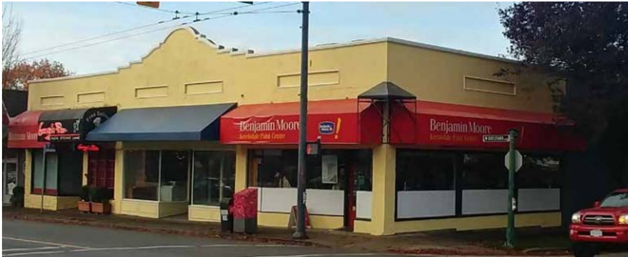
East elevation (left) and north elevation (right) of the S.E.P. Block (2019)
