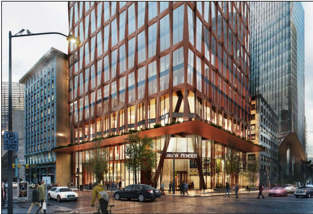
Figure 4 – View of the Ground Floor at West Pender and Seymour Streets
