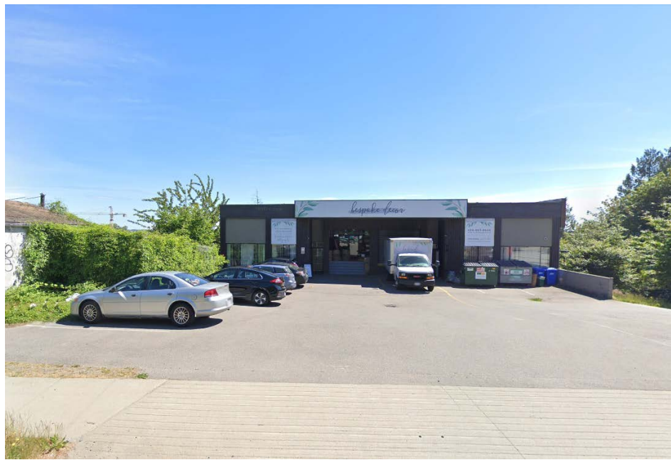
Existing two-storey industrial building
